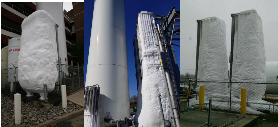
Vaporizers that are more than 50% iced (contact Airgas)
